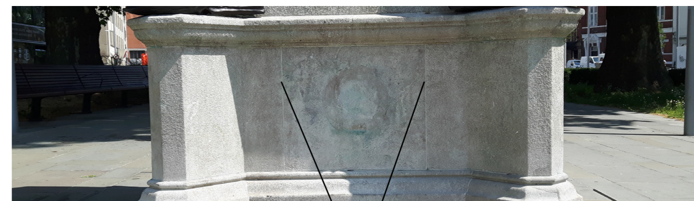
Mortar joints on pedestal
